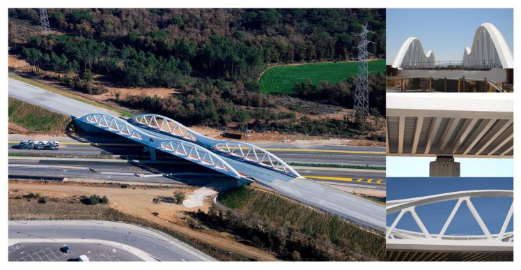
The structure consists of a single two span deck of 53.0m + 53.0m between axes giving a total length of 106.0m. The structure has a marked skew and therefore the axis supports on the piers and abutments offer an angle of 34.3° on the high speed train line. The width of the deck is a constant 15.70m.
